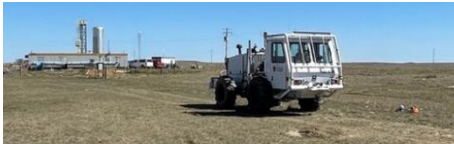
Figure 6. Vibroseis surveys along the fibre optic trench at CaMi FRS.
