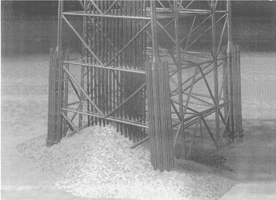
Figure 3: Graphical representation of a platform jacket and cuttings pile (Heather Platform) courtesy of AEA Technology
