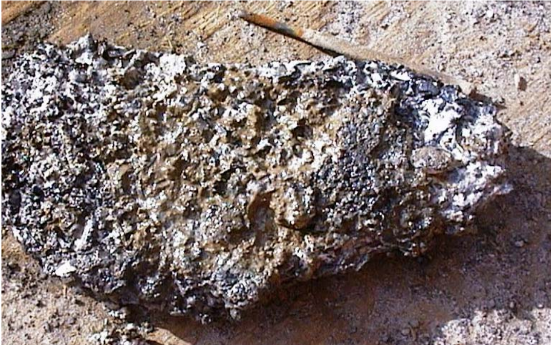
Figure 56: A closer look at a piece of the crust from the Ekofisk 2/4 A.
