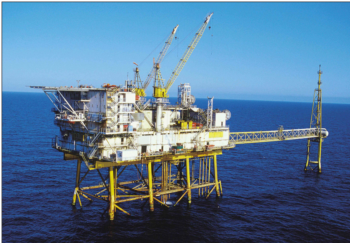
Figur 3.14. Plattform COD 7/11. Foto: Phillips Petroleum Company Norway/Kjetil Alsvik
