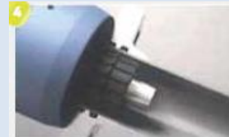
4 Tool removed and flange ready.
