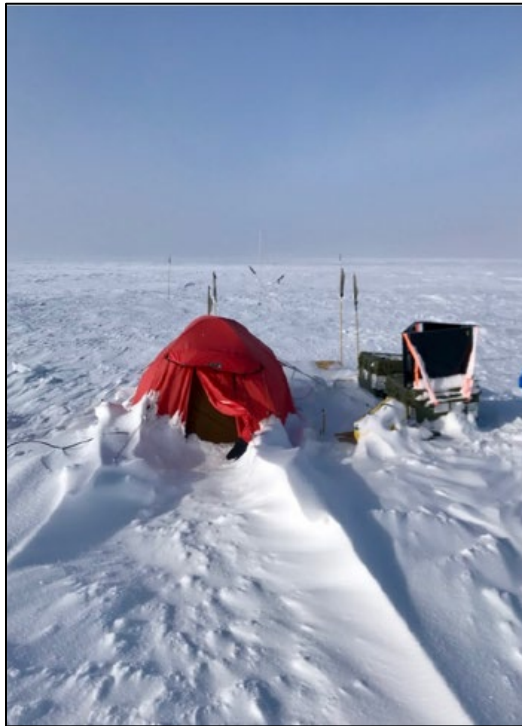
Figure 8: The field setup at the Skytrain Ice Rise. The interrogator is housed in the tent and powered by a petrol generator located 50m away. The large green Pelican Case houses the DTS equipment, which is powered by the solar panels. Over 600m of cable is deployed in a vertical borehole marked by the flag behind the Pelican Case
