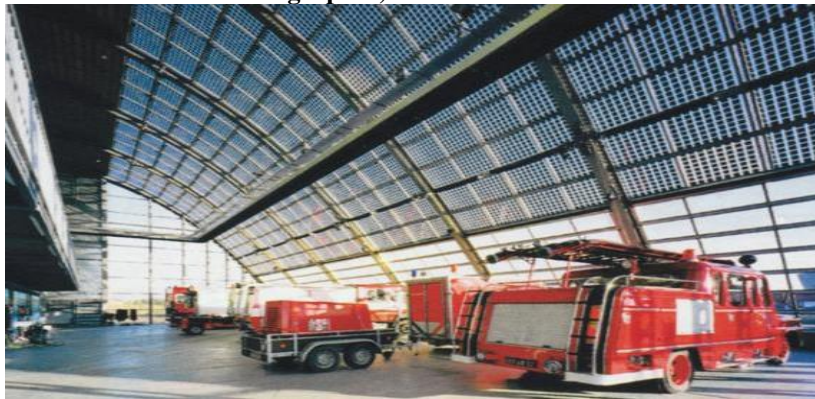
Figure 31: Fire station in Houten, Netherlands, designed by Philippe Samyn. (Source: Novem, Hans Pattist).
