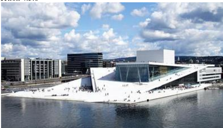
Figure 35: The new opera house in Oslo. Solar cells are integrated in the triangular, south facing glass façade. Kilde: [Fornybar, 2010].
