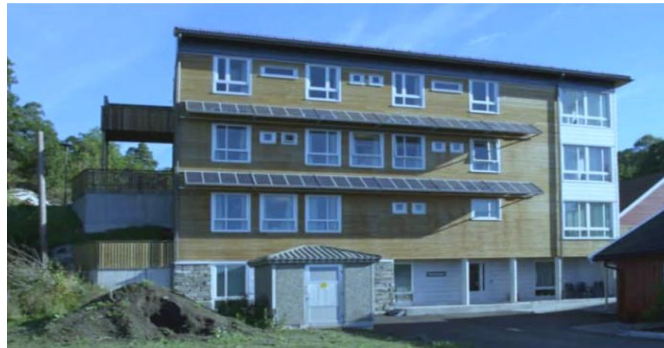
Figure 49: Kongsgaard Rehabilitation Centre, Kristiansand – PV sunshades.
