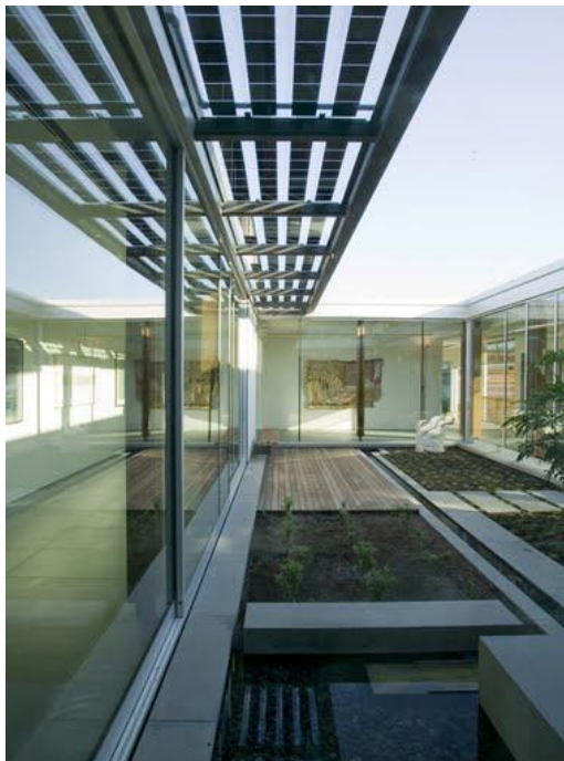
Figure 44: Sun screening of window by solar cells from Atlantis Energy Systems ( http://atlantisenergy.com ).
