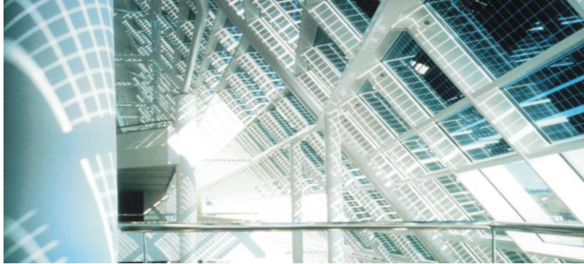
Figure 30: The inside of Solar Office Doxford International, Sunderland, UK. (Source: Denis Gilbert Photographer).
