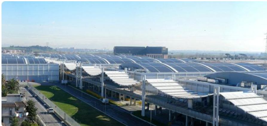
Figure 47: Rome Trade Fair in Italy has 1400 kW PV installed. The modules are flexible thin film panels from UNI-SOLAR. Source: www.uni-solar.com .
