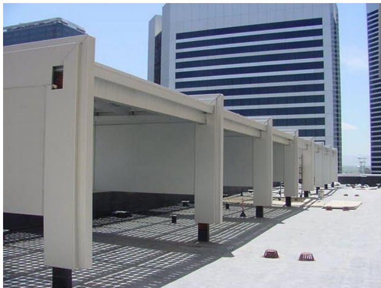
Figure 43: Shading of parking lot with semi-transparent PV modules, from Atlantis Energy Systems ( http://atlantisenergy.com ).
