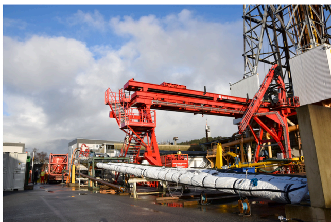
Fig. 1. View of the four test assemblies draped in insulation and plastic covers.
