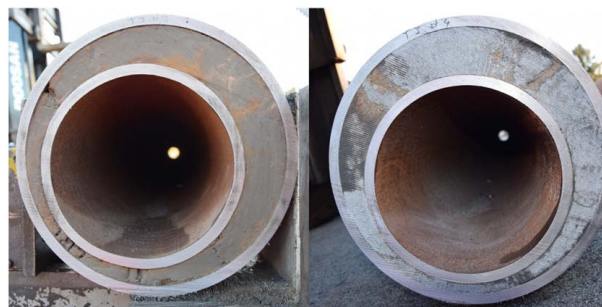
Fig. 4 Exposed top (left) and bottom (right) of the transition joint
